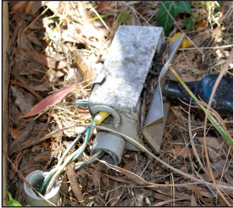
Typical electrical/system boxes are vulnerable to breakage and weather wear.
